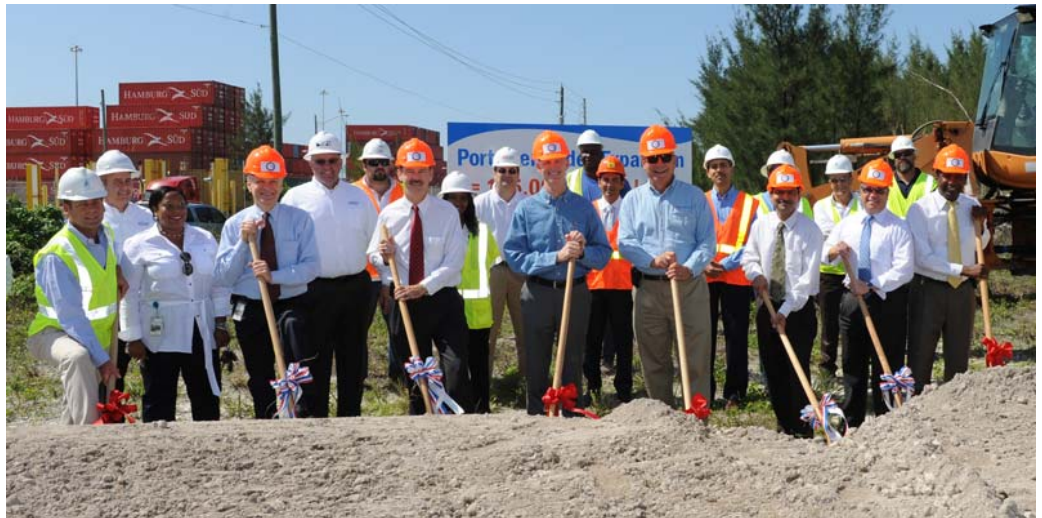
Ground breaking ceremony on Eller Drive Overpass with Florida Governor Rick Scott.
